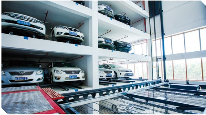
立體型 [原圖來源：深圳怡豐自動化科技有限公司] Vertical lifting and horizontal sliding system [Source of the original photo: Shenzhen Yeefung Automation Technology Co. Ltd.]
