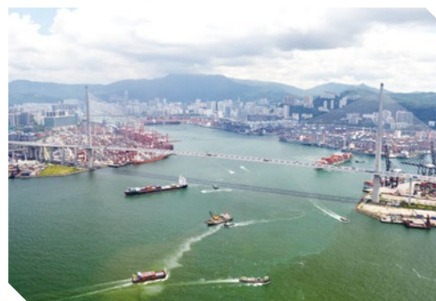
昂船洲大橋 Stonecutters Bridge
