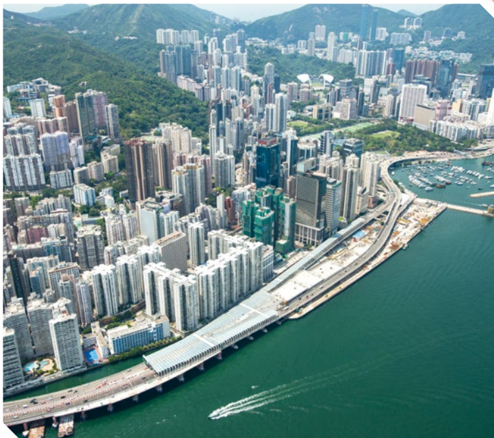
中環及灣仔繞道接連東區走廊鳥瞰圖 The Central-Wan Chai Bypass links up with the Island Eastern Corridor – an aerial view
