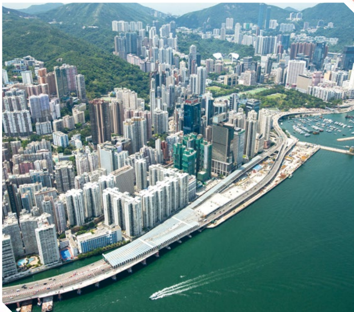
中環及灣仔繞道接連東區走廊鳥瞰圖 The Central-Wan Chai Bypass links up with the Island Eastern Corridor – an aerial view
