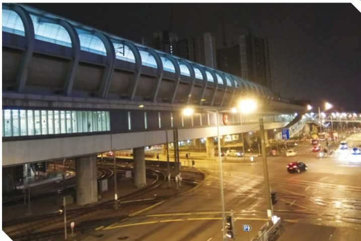
西鐵天水圍站 Tin Shui Wai Station on the West Rail Line
