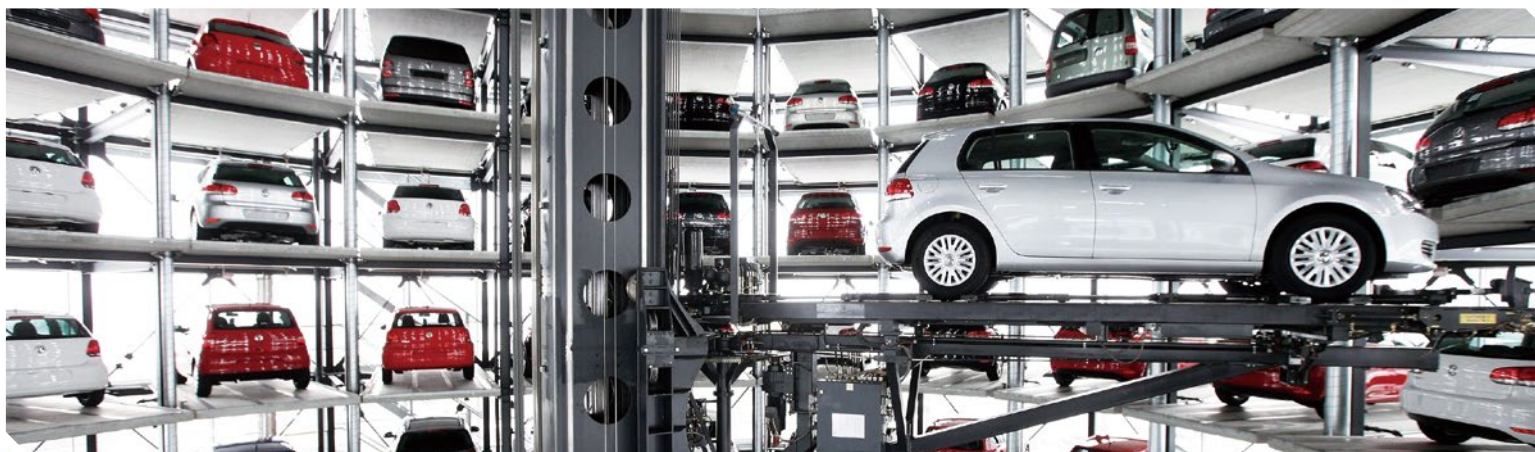
圓筒型 [原圖來源：Autostadt GmbH, Germany] Circular shaft lifting system [Source of the original photo: Autostadt GmbH, Germany]
