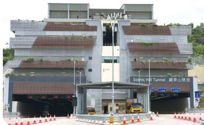
觀景山隧道 Scenic Hill Tunnel
