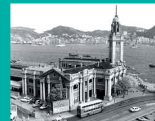
尖沙咀鐘樓前身為九廣鐵路香港段的總站 The Clock Tower in Tsim Sha Tsui was once the terminus of the Kowloon-Canton Railway (Hong Kong Section)
