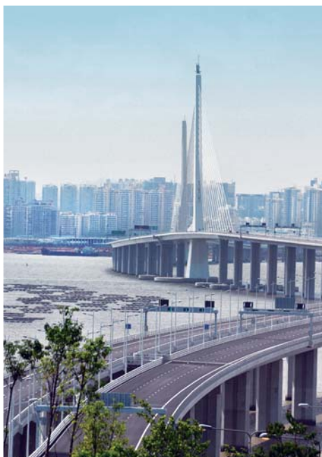
深圳灣公路大橋連接新界西北及深圳蛇口 Shenzhen Bay Bridge connects northwest of Hong Kong with Shekou, Shenzhen
