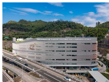
Transport Department Vehicle Examination Complex
