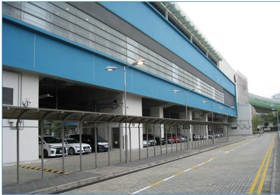
Ocean Park Station Park and Ride Facilities
