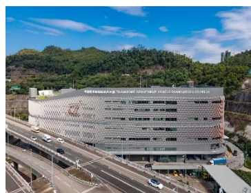
Transport Department Vehicle Examination Complex
