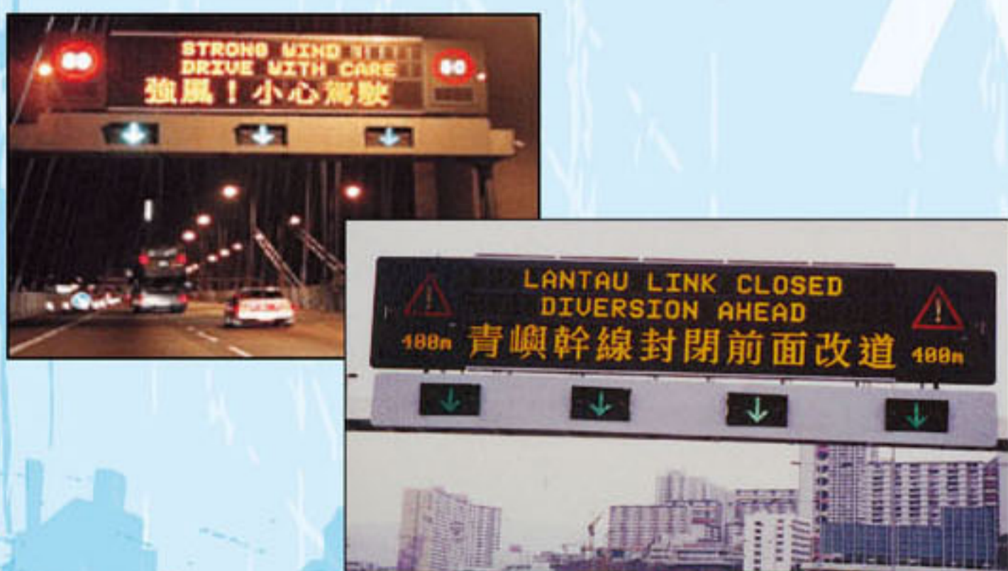
青馬管制區的交通管制及監察系統 Comprehensive traffic control and surveillance system at the Tsing Ma Control Area
