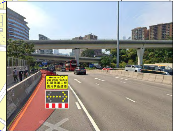
漆咸道北 (西行) Chatham Road North (Westbound)
