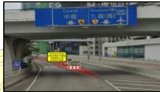
干諾道天橋 (東行) Connaught Road Flyover (Eastbound)
