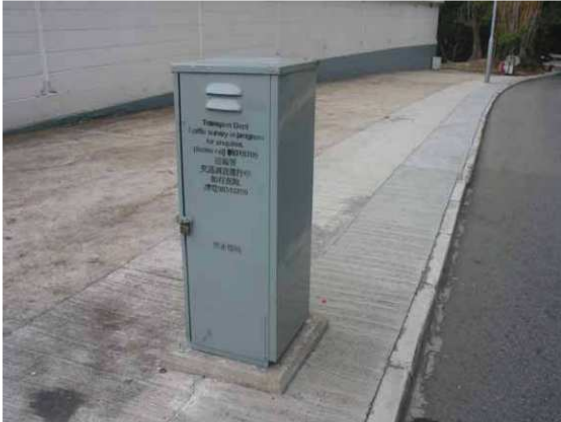
ATC Loop and Roadside Cabinet
