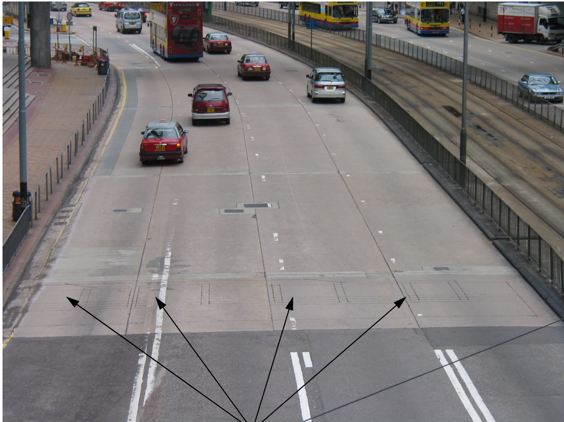
Loop Detector installed in concrete slab
