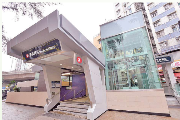
接驳路面及港铁车站大堂的升降机 External lift connecting street level to concourse
