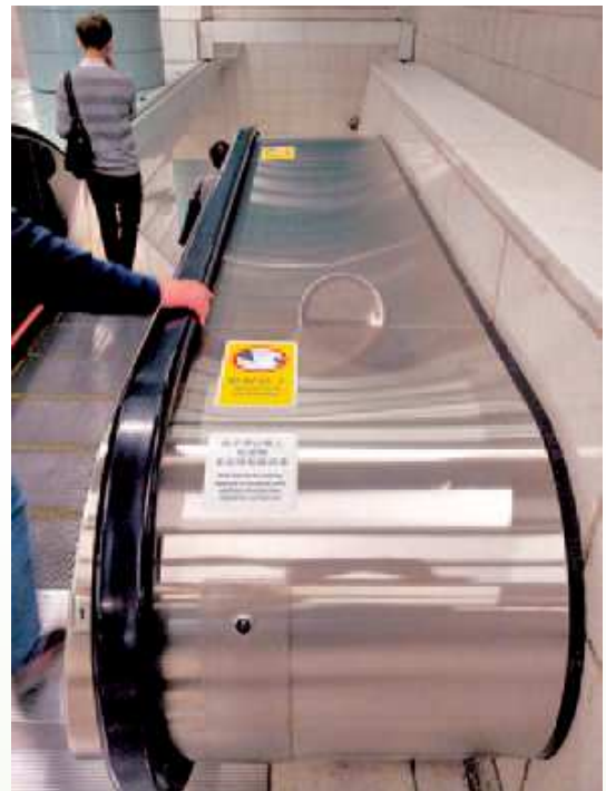
扶手电梯附设发声器 Audible device at escalators
