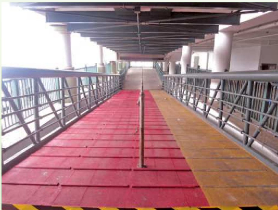
铺有防滑物料及设有槽纹的码头斜道 Ramps with anti-skid gangplanks and grooves at pier
