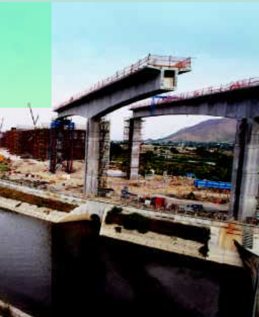
錦田附近的西鐵工程。 West Rail under construction near Kam Tin.
