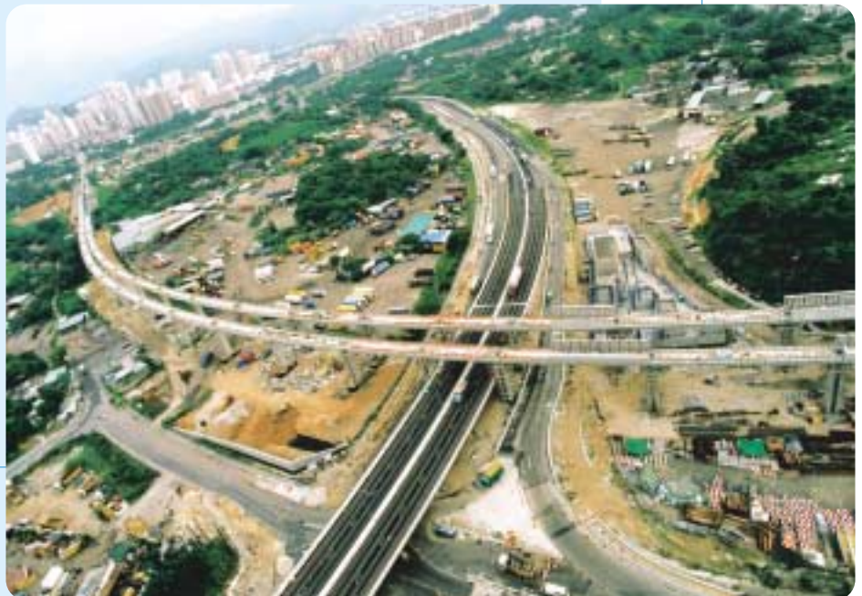
建於新設天水圍朗天路天橋上的西鐵高架路。 West Rail viaduct above a newly-completed flyover over Long Tin Road at Tin Shui Wai.
