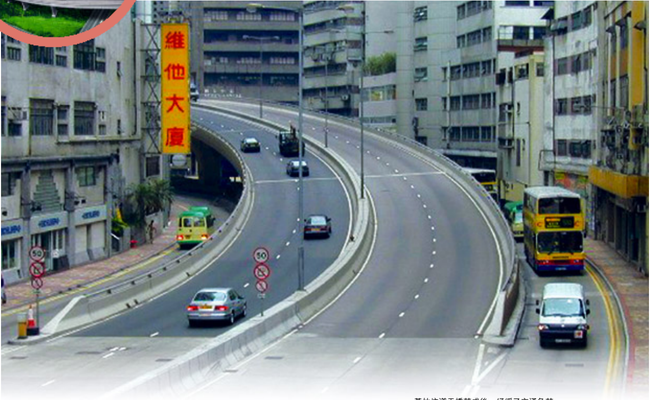
黃竹坑道天橋落成後，舒緩了交通負荷。 Completed Wong Chuk Hang Road Flyover improves traffic flow.
